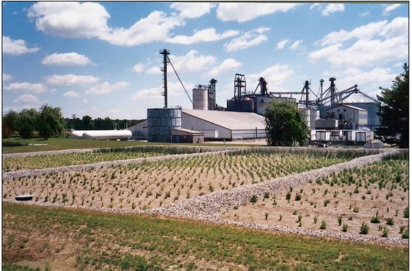
Rose Acre Farms installed both wastewater and storm water constructed wetlands to provide environmentally sound water treatment, while reducing operating and maintenance costs. (Shown above: Rose Acre Farms several days after project was completed)
