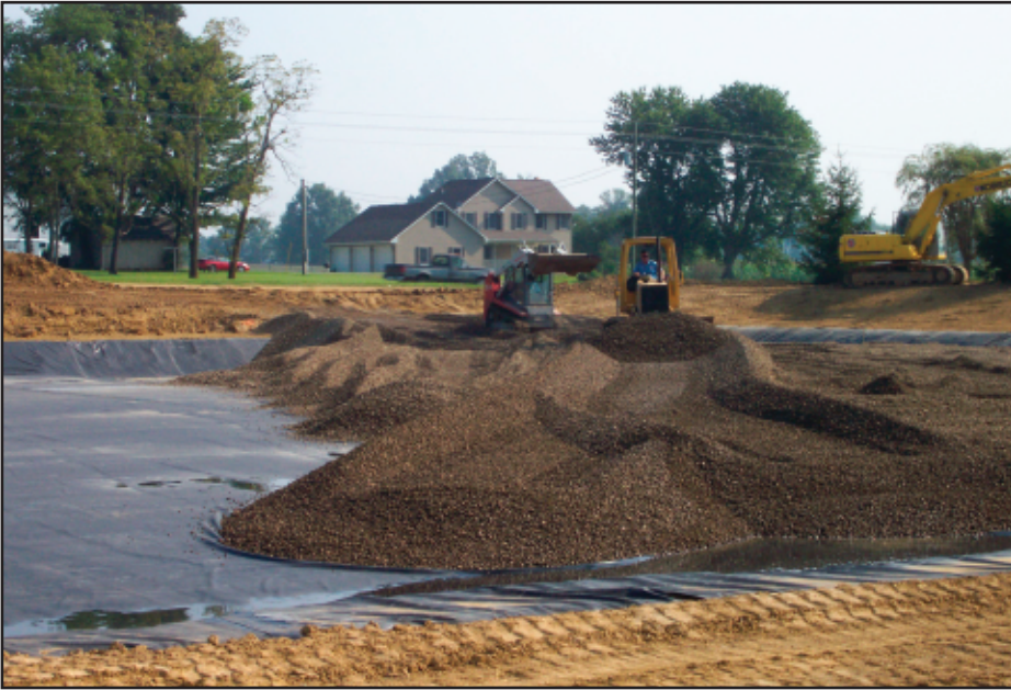
After minimal training from a company representative, Rose Acre Farms was able to install the liner themselves.
